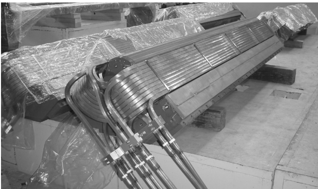
Fig. 4, New QC2 coils made of MIC mounted on the existing iron yoke. Old QC2 coils insulated by epoxy were removed and stored for future recirculation.
